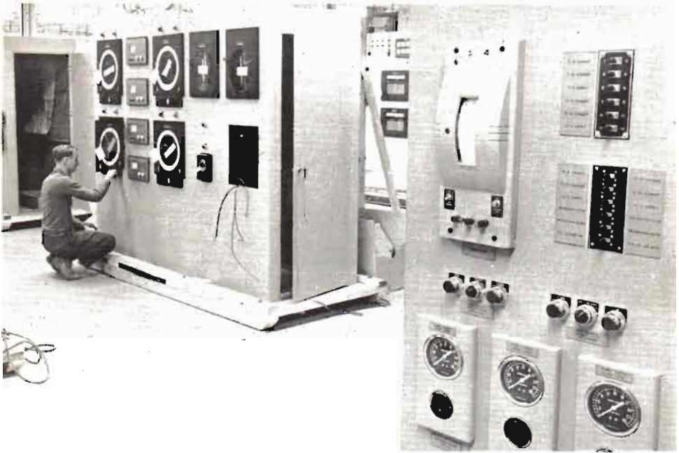
Panel Shop—Honeywell Controls Limited, Scarborough, Ontario
